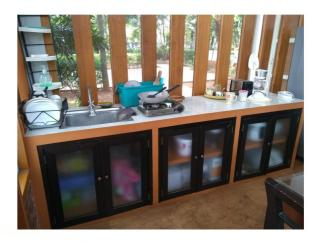
This Kitchen Table is made from lightweight concrete and it has door from aluminium and glass.
